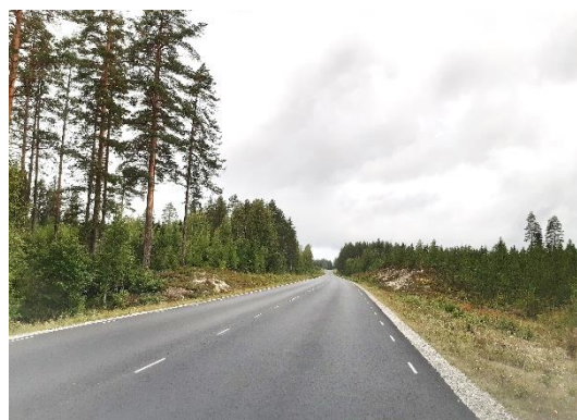
Figure SEQ Figure \* ARABIC 2 Newly renovated road no. 518 between Eno and Kyyrönlampi. This is the main route connecting Lieksa with Joensuu.
